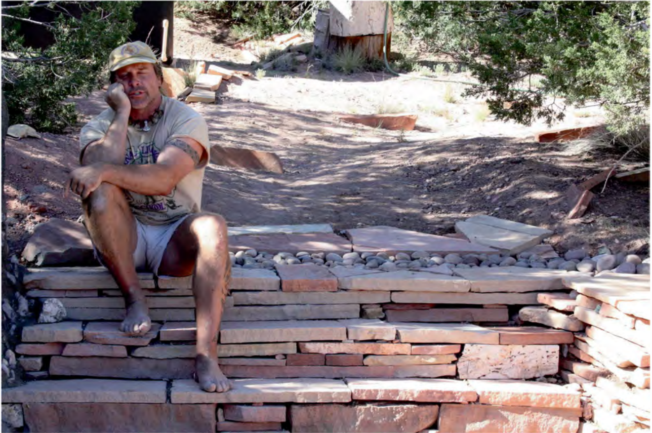
CODY LUNDIN APPRECIATING THE NEW STEPS WE BUILT WHICH INCORPORATED A "DRY CREEKBED" LEADING RAINWATER TO A NEARBY PLANTER RETAINING WALL TO TAKE CARE OF AN ERROSION ISSUE.
